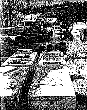
Once tanks are set, on-site SeptiTech technicians complete system installation.
